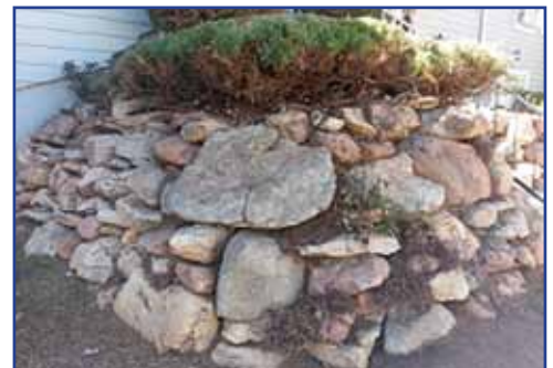
CH Board and Landscaping Committee members trimmed bushes, cleaned grassy areas, and trimmed juniper bush to expose rock retaining wall.
